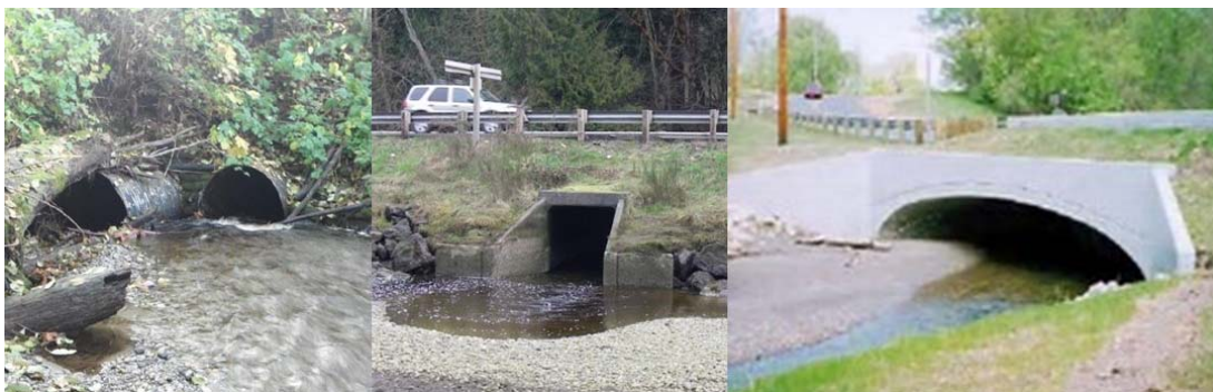
Existing culverts at 144 th Street NW and SR 302 Proposed new culvert concept
