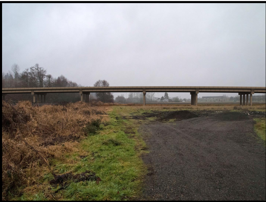
Proposed, looking west from a residence toward BNSF Railway.
