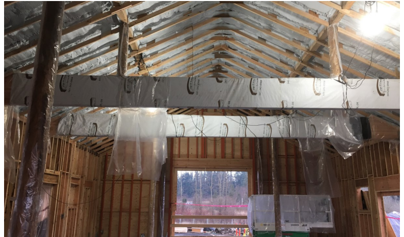
SPRAY FOAM INSULATION AT UNDERSIDE OF CEILING
