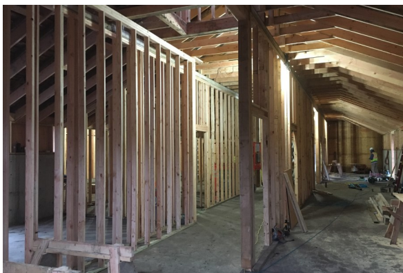
INTERIOR FRAMING NEAR COMPLETION
